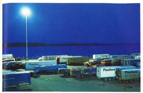
Pandoro's security-bonded compound at Fleetwood Docks is floodlit by 400W Solarcolour Plus lamps in Eurofloods mounted on high mast columns,
