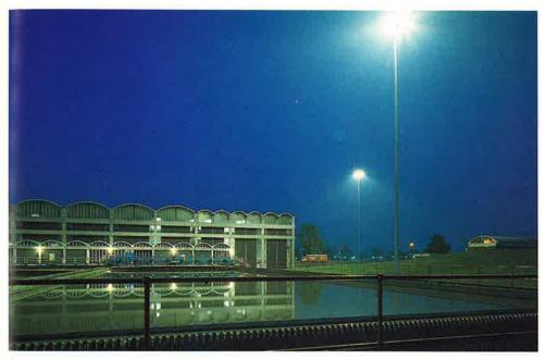
GEC Spacelight lanterns with 400W SON-T lamps are mounted on 30 metre masts to floodlight Strathclyde Regional Council Shieldhall Sewage Works in Glasgow.
